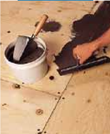
Grouting of plywood substrate with Nivorapid + Latex Plus
